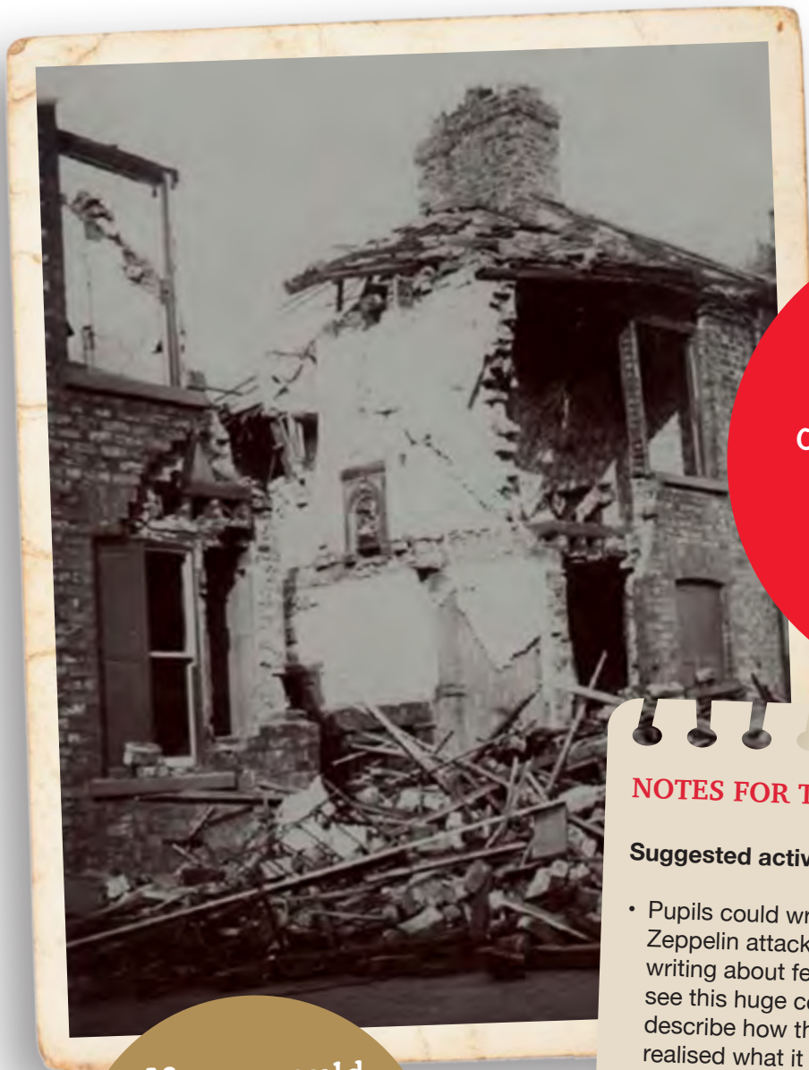
Zeppelin damage in Kyme Street, Bishophill
